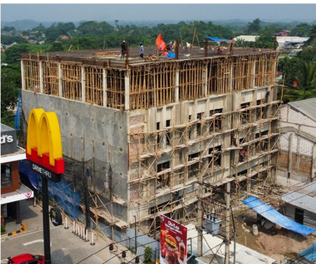
Cisauk, BSD Shophouse Project
