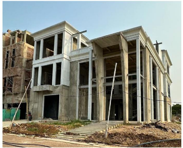
Palm Spring Boulevard - PIK 2 Building Structure
